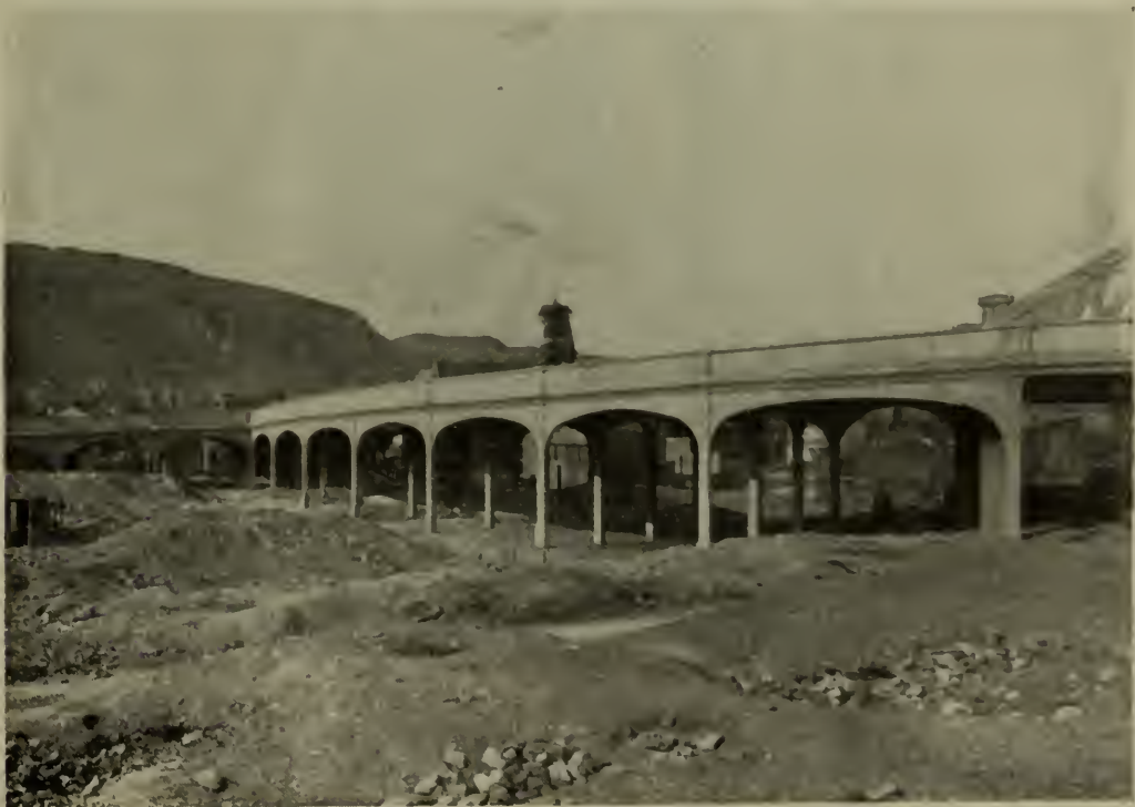
FIG. 1. PART OF VIADUCT AND SPUR VIADUCT.
